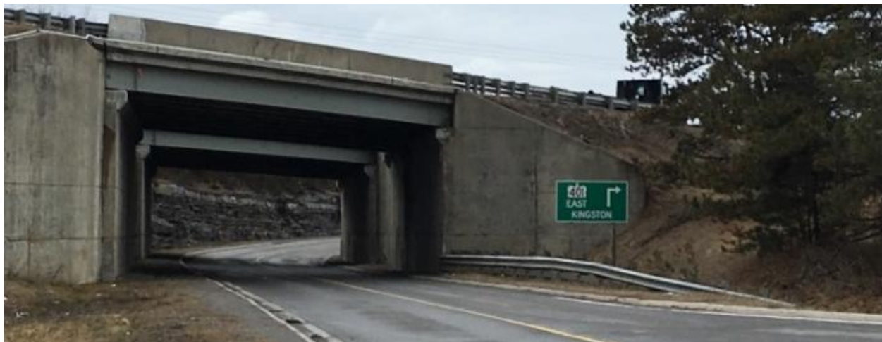
Figure 4-8: Overpass – Palace Road at Highway 401
