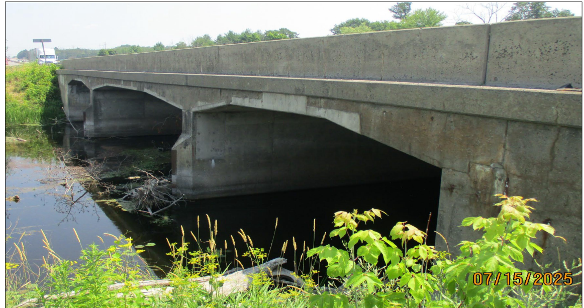
Existing Napanee River Bridge
